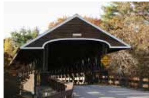
Rowell Covered Bridge
