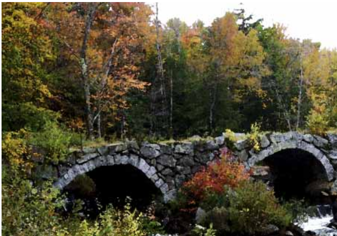
Stoddard Fall Stone Bridge W/C
