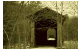
Kellyville RR bridge
