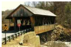
Packard Hill Bridge
