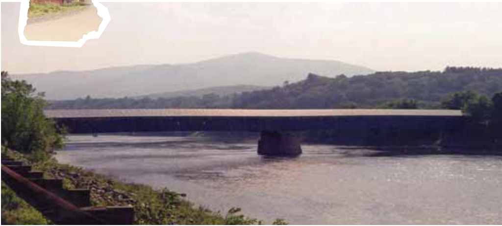
Cornish Windsor Bridge
