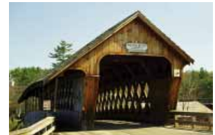
Squam River Bridge
