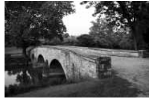
Burnside Bridge B&W
