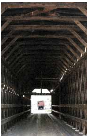
Bridge in time w/c
