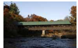
Rowell Covered Bridge w/c
