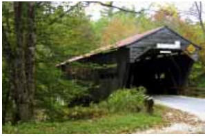
Durgin Bridge W/C
